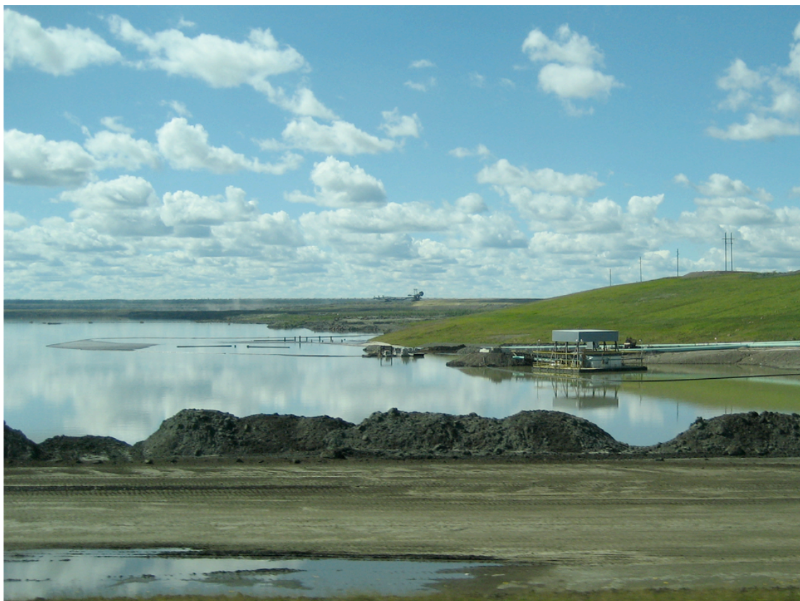
Figure 21. Syncrude Tailings Pond West of Highway 63, which will become an end pit lake. Note water treatment facility in midground and bucketwheel reclaimer in background. Dark mounds in foreground are low-grade oil sands. (MTW, 20 August 2006)
