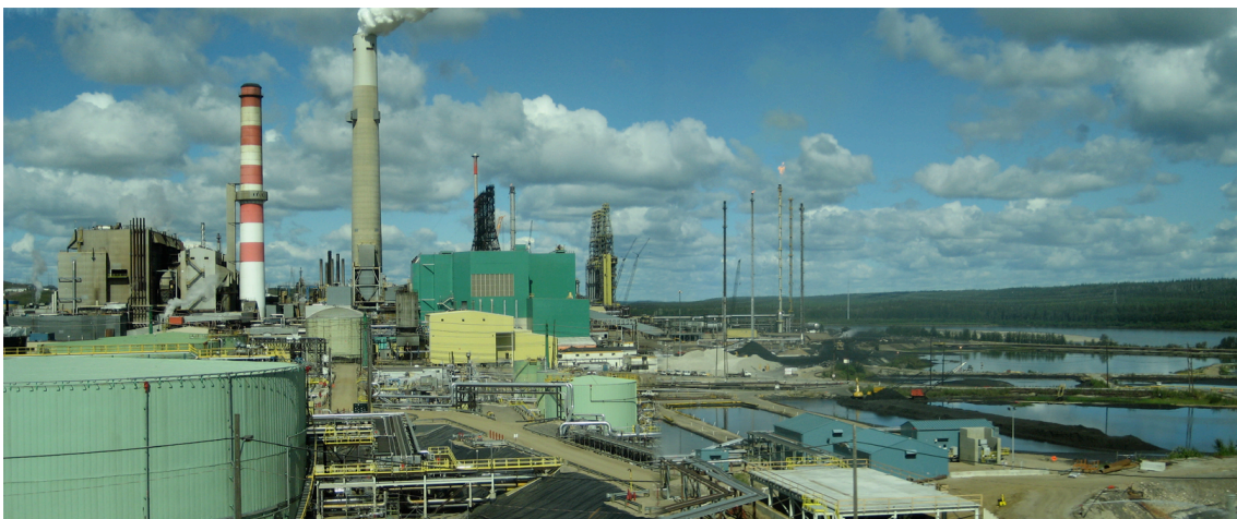
Figure 14. Panorama of Suncor plant. Note holding tank and power plant at left, upgraders in middle, and settling basins next to the Athabasca River at right. (MTW 20 August 2006)
